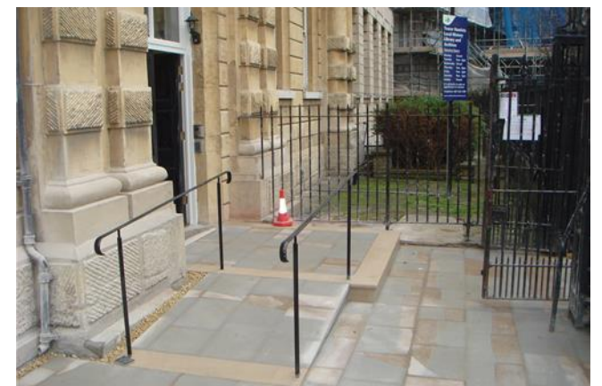
New entrance ramp, step and power-assisted doors
