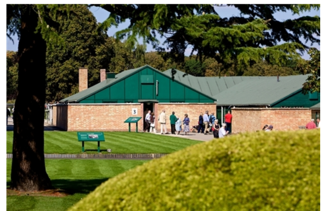
Restored wartime huts. Car parking was removed from the historic parkland and lawns were re-laid. The blast walls were reinstated to match historic images. Colours were analysed and reproduced
