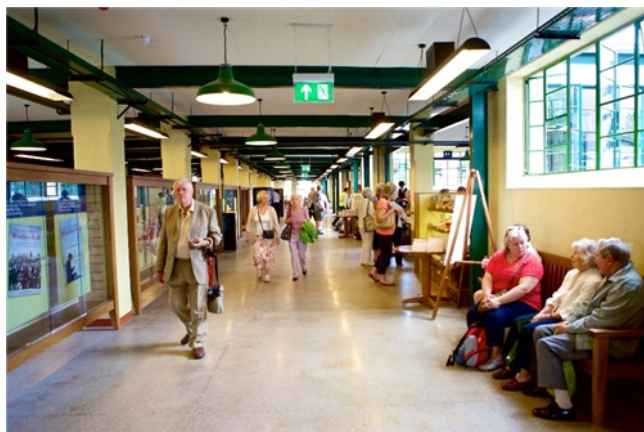
Spatial divisions were defined by showcases to preserve the integrity of the open-plan computer hall, with designs based on the WWII filing cabinets. Original acoustic ceiling tiles were treated for fire resistance and re-instated
